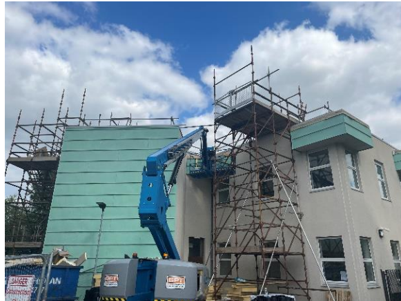
Ongoing EEDPP upgrade of the Burrin Building, Kilkenny Road Campus
